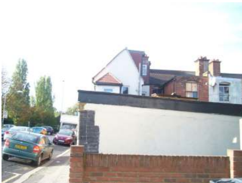
Showing rear elevation of existing garage that is proposed to be demolished. With an erection of new self contained studio flat in similar size and scale.
